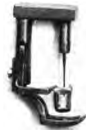
Fig. 3. Guard for Needle of Sewing Machine. (Pat.)
